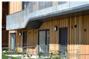
Clyde Valley Housing Association Coatbridge Library, Coatbridge
