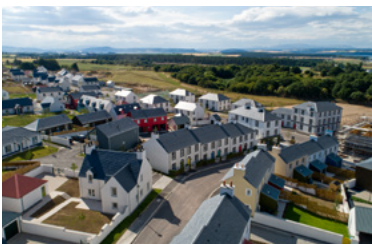
A & J Stephen (Builders) & ZeroC Holdings Phase 1A, Tornagrain
